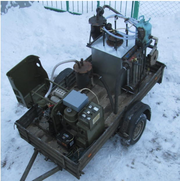
Fig. 3. General view of the gas generator
